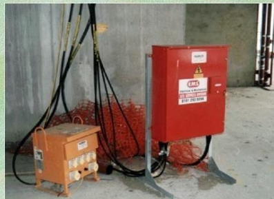
Rising Main Unit and Transformer
