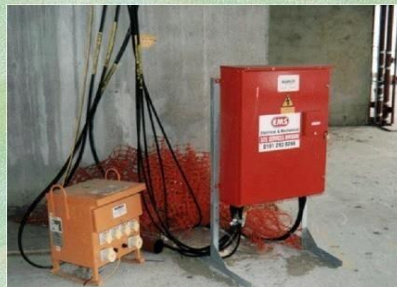
Rising Main Unit and Transformer
