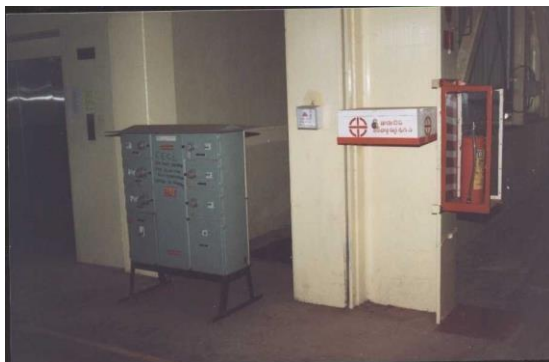
Rising Main Unit and Transformer
