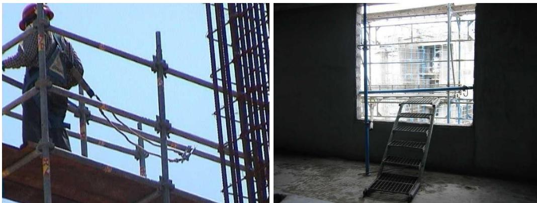
Full body harness with double lanyard Proper Access to work platform
