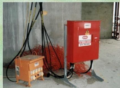
Rising Main Unit and Transformer
